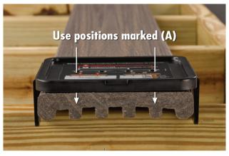
Install screws in positions marked A to ensure proper placement centered in the scalloped profile for standard installation
